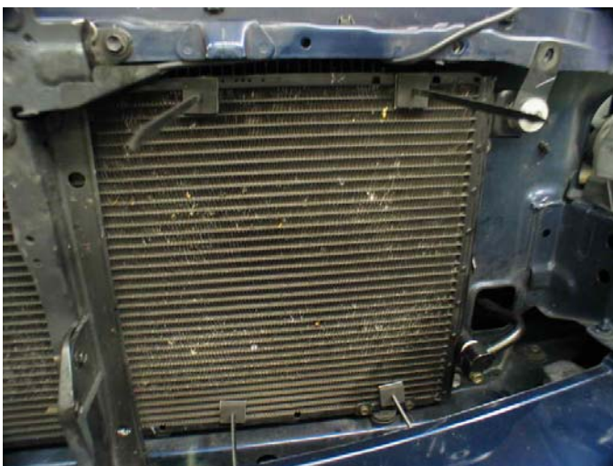
Picture 5. Nylon straps protruding through the condenser fins with foam pads installed. The condenser hardware has been reinstalled, sans the horn on the right side of the core support.
